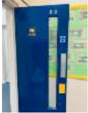
Good vision panels and all doors have been numbered.
